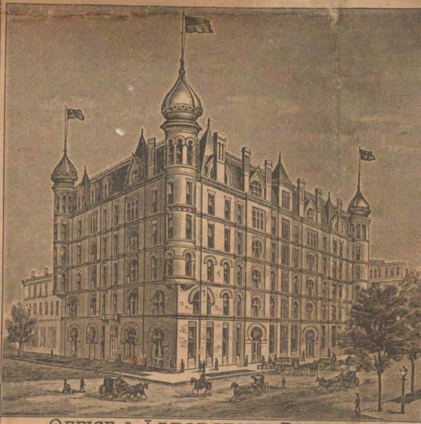
OFFICE & LABORATORY BUILDING H.E. BUCKLEN & CO. CHICAGO, ILL.
