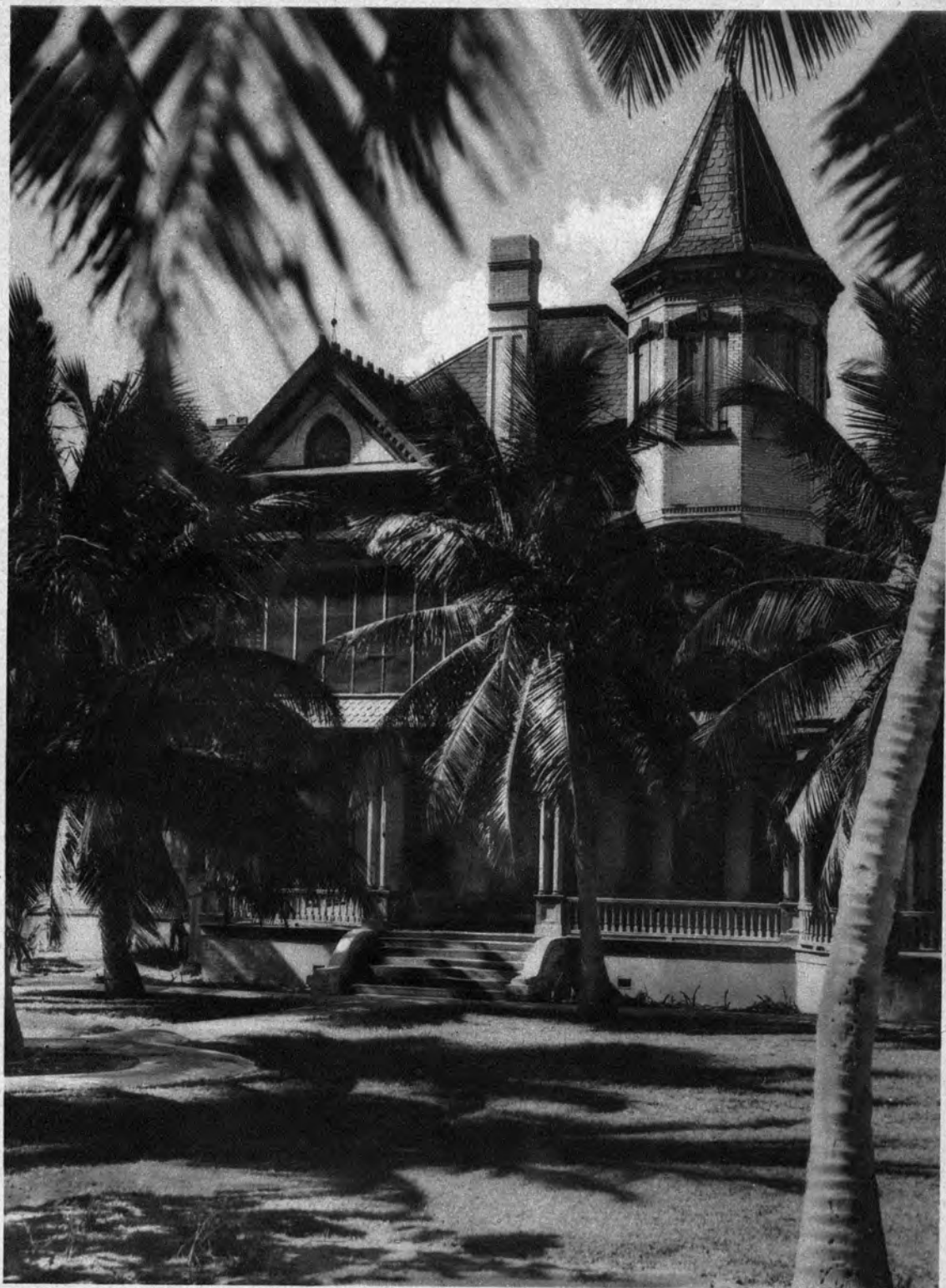
The house pictured in the above photograph is built on the southernmost piece of land in the United States and is rightly called t h e SOUTHERNMOST HOME.
