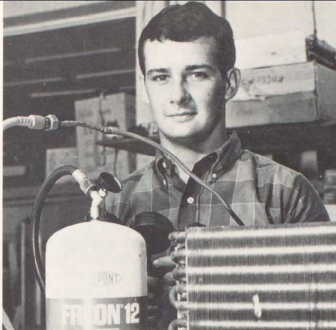
Lee Norris trains in air conditioning at Summerland Electric.
