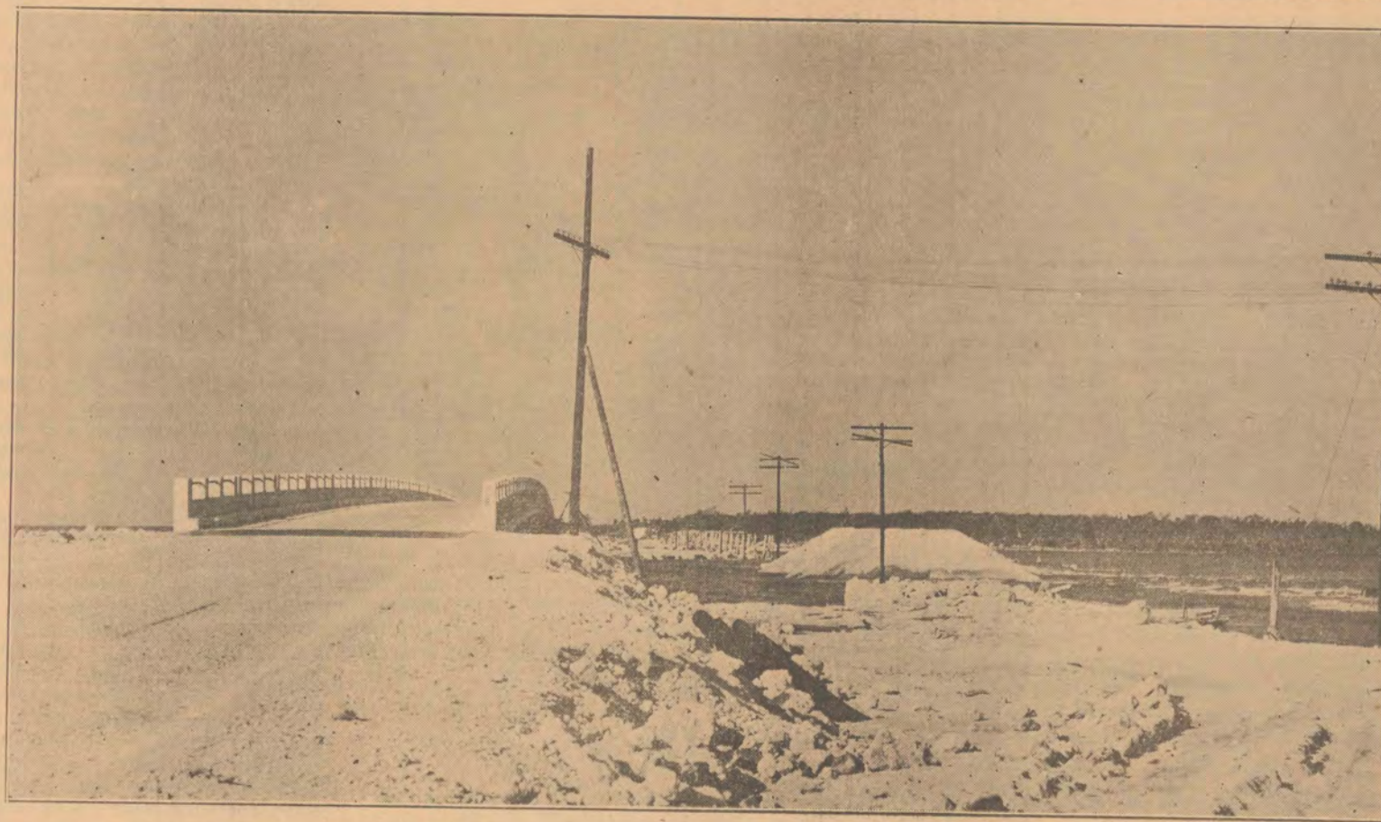
CONSTRUCTION ON LOWER MATECUMBE
