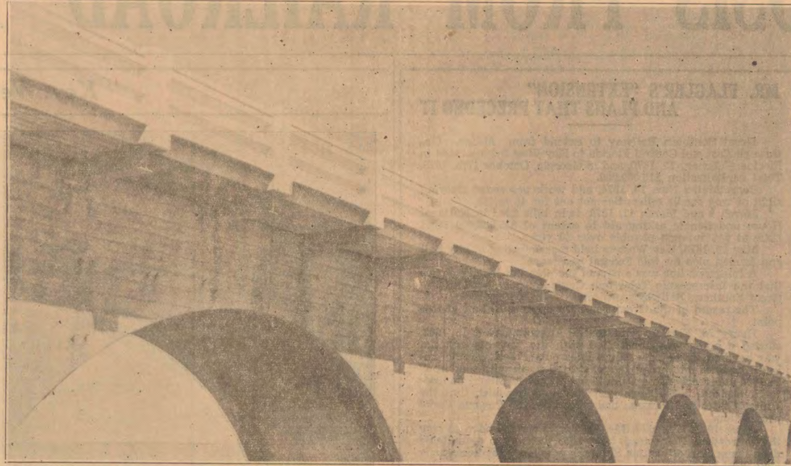
ROAD CONSTRUCTION OVER ARCHES
