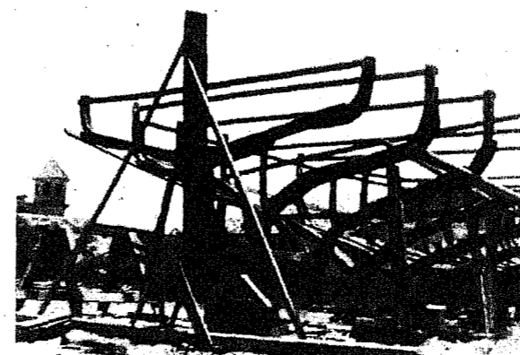
One-third of the ribs in place as the hull was being laid.
