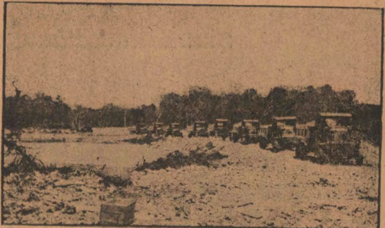
Hundreds of tons of fill being brought to the Matecumbe road pro- ject in Jenner Bros.' fleet of trucks.
