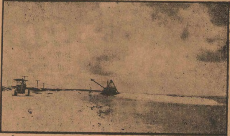
The roller putting the finishing touches to the Matecumbe fill mak- ing it ready for the tourist along the Keys.
