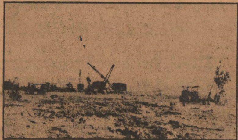
Showing the dredges, shovel, scraper and roller at work on a sec- tion of the big fill at Matecumbe.
