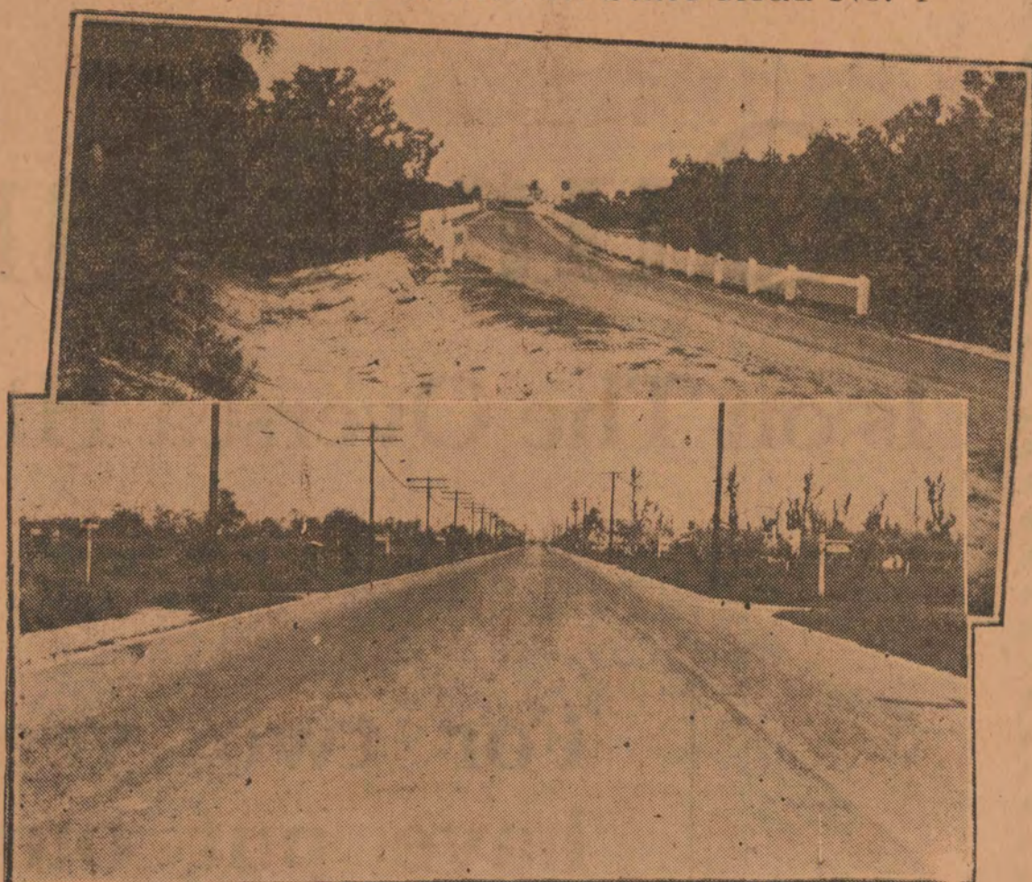
Top—One of the well rounded curves and the guard fences which are constructed as an added safety feature. Bottom—A straight-of-way in the link of No. 4 in St. Johns and Flagler counties.
