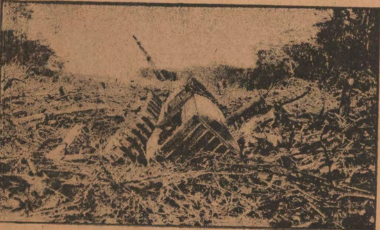
This big caterpillar tractor was nearly lost in the mangrove swamps in the early stages of the highway work as the way was cleared for the present splendid roadway.
