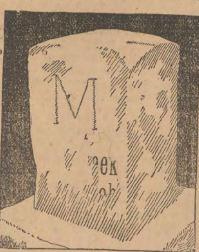
Marks a Boundary Line.
