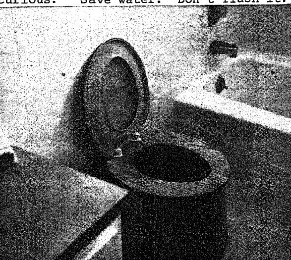
The waterless Clivas Multtrum toilet, the basis of the house's waste disposal system.
