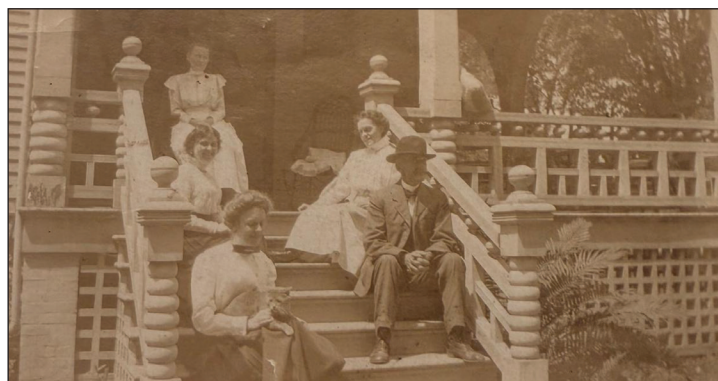
THIS 1911 PHOTOGRAPH shows the Fenelon family on the front porch of their house at 404 Ransom St. Pictured are, clockwise, from bottom left, Daisy Fenelon, Violet N., Ophelia (Lilia) Bloom Fenelon, Lillian Fenelon and John E. Fenelon. The house was demolished in 1969.
