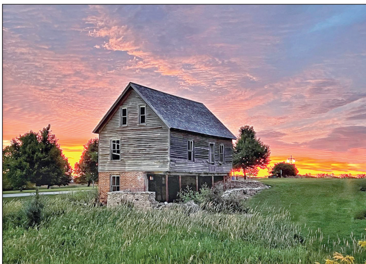
THIS BUILDING OFF Douglas Street in Riggs County Park recently was razed. It was the last farm building connecting the land to its history as the Sherwood farm, which remained in the Sherwood family from 1866 until 1998. Al Klapperich photo
