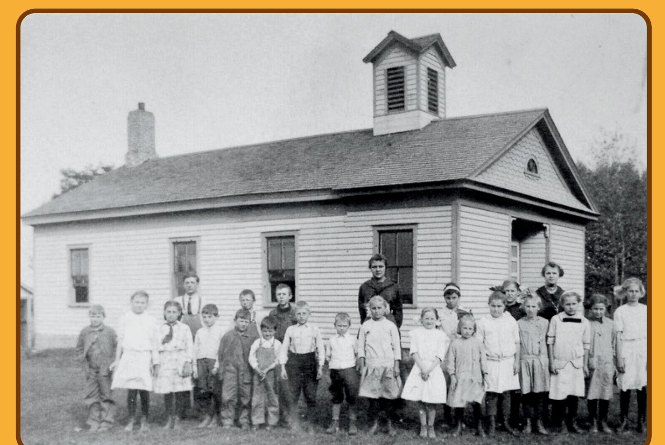
Adams School, 1851 Located, Hwy 23E
