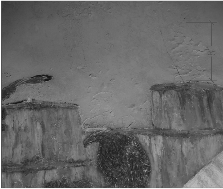
West elevation: note poor condition of mural surface at select areas of sky/ horizon. Photo digitally enhanced.
