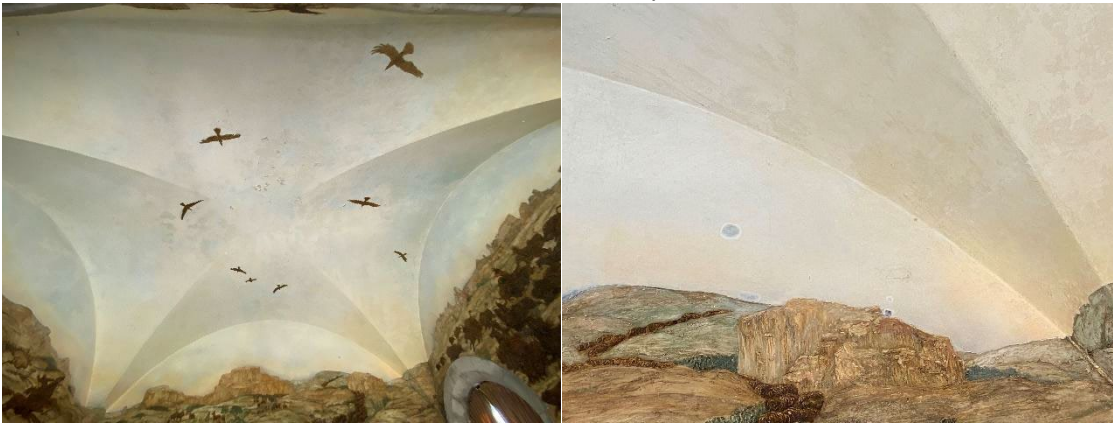
Ceiling shared by client
