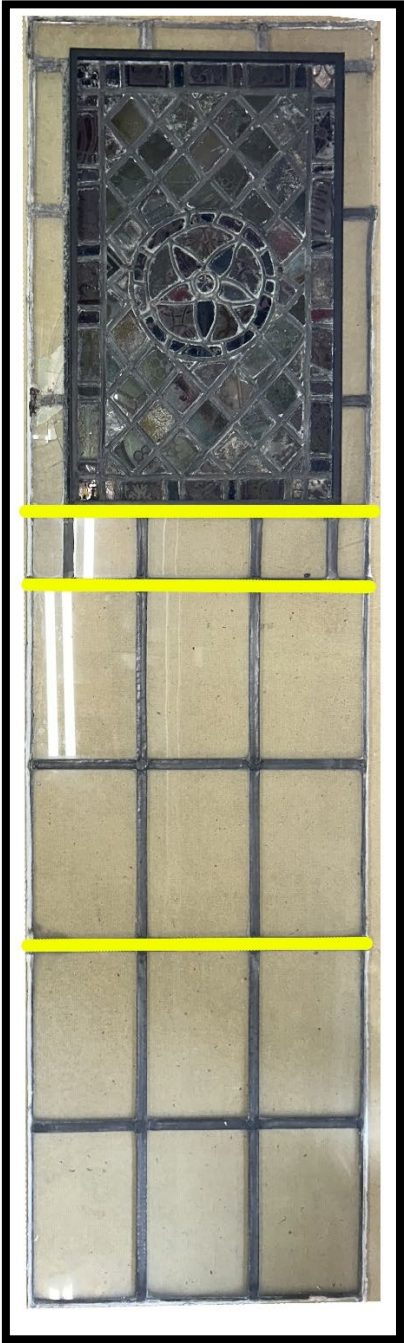
FIGURES 11 and 12: Existing conditions diagrams, broken glass for replacement (left) and hollow heart lead came (right)
