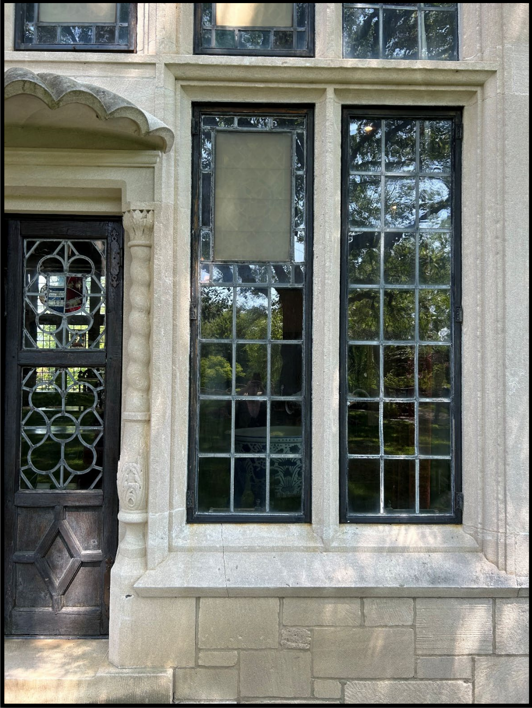
FIGURE 2: Exterior view on site, before conservation
