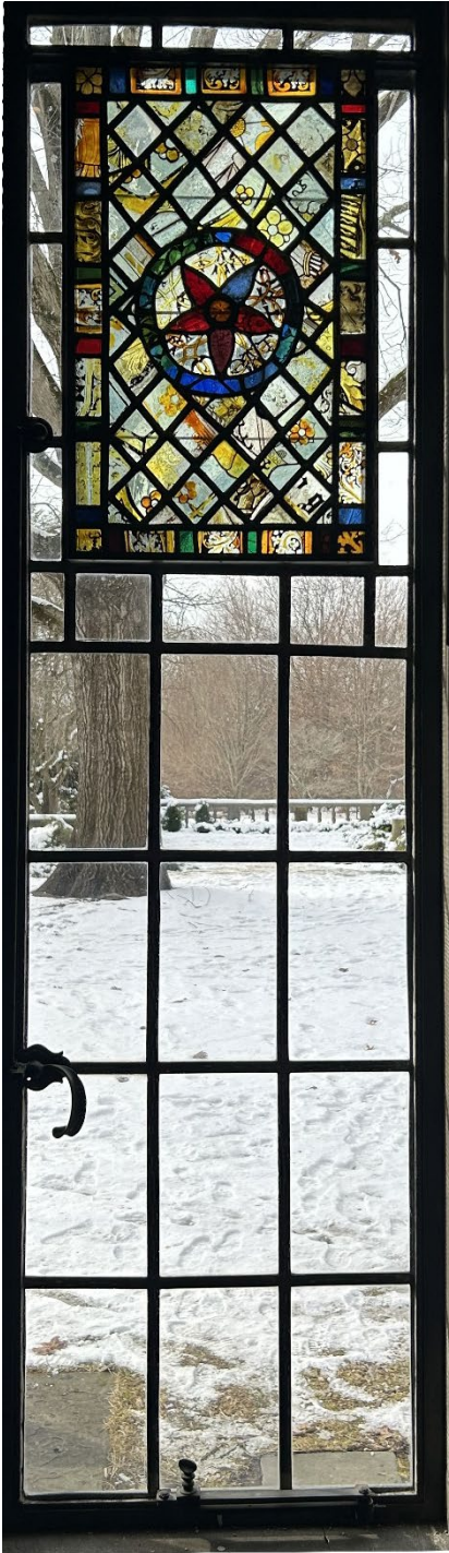
FIGURE 18: Finished panel reinserted on site, interior view
