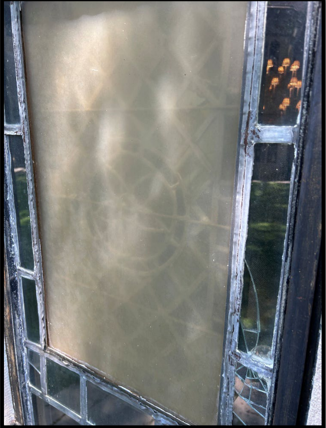
FIGURE 4: Detailed views of broken glass and yellowed Lexan panel
