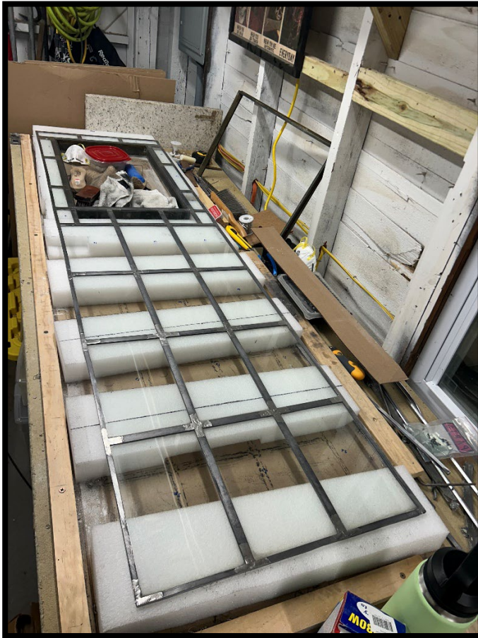
FIGURE 15: Re-leaded panel with new comes, exterior and interior views
