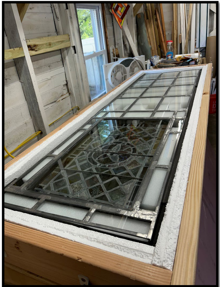
FIGURE 16: Historic panel reinserted into window and packed in box for transport
