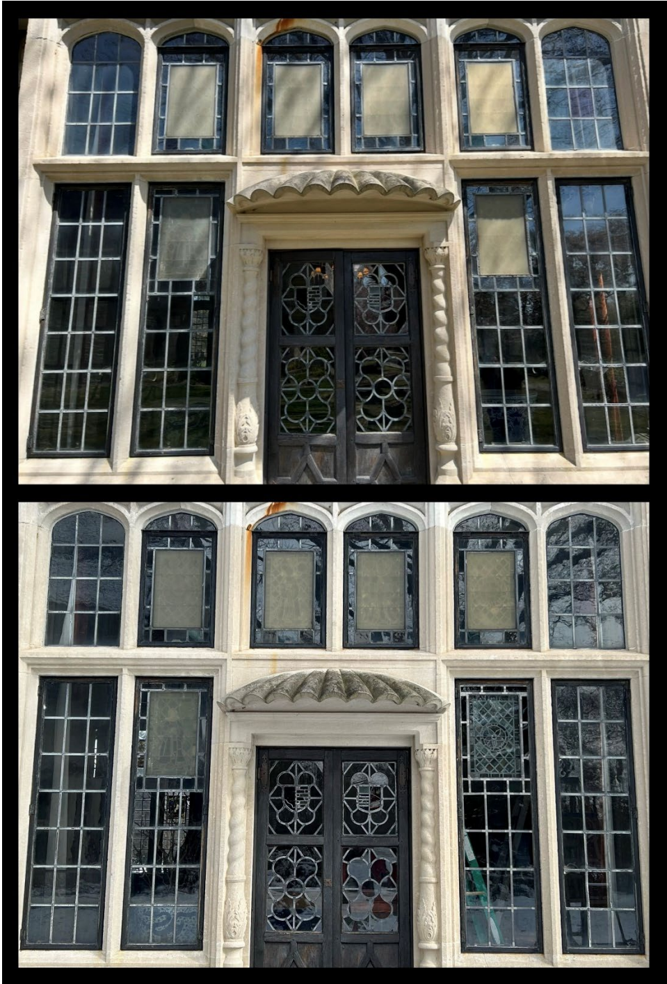
FIGURE 22: Before and After conservation, exterior view
