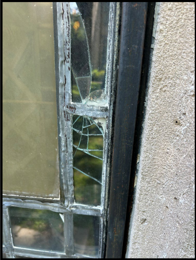
FIGURE 4: Detailed views of broken glass and yellowed Lexan panel
