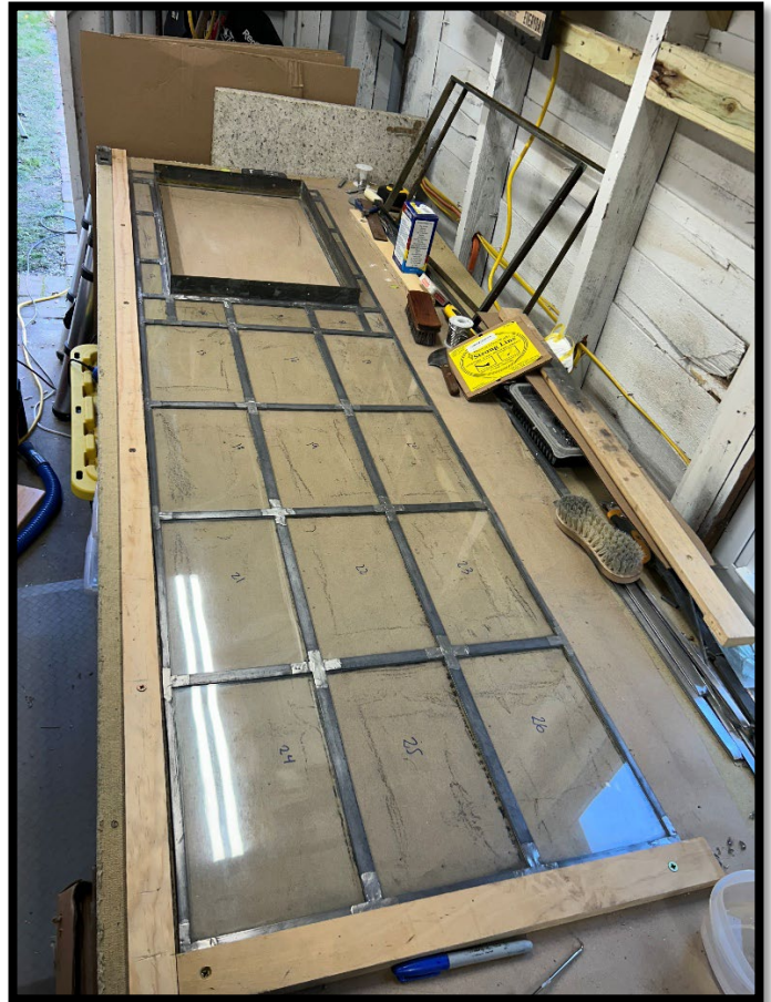
FIGURE 15: Re-leaded panel with new comes, exterior and interior views
