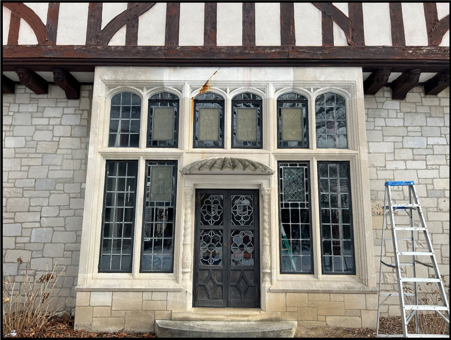
FIGURE 17: Finished panel reinserted on site, exterior view
