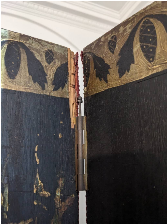
Losses & Loose Pin, Middle Top Section
