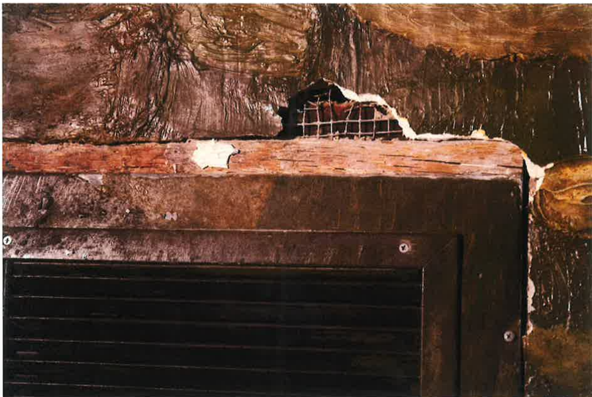
South Elevation - Approximate Grid Location #4
