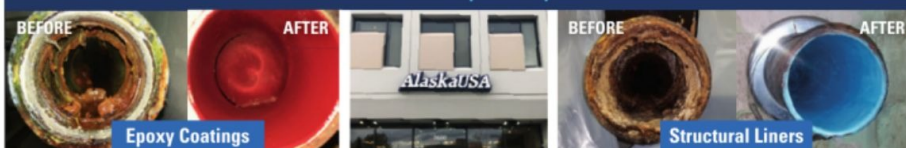
3" Water Main Before & After Epoxy Coated
