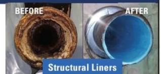
6" Cast Iron Drain Line Before & After Epoxy Lined
