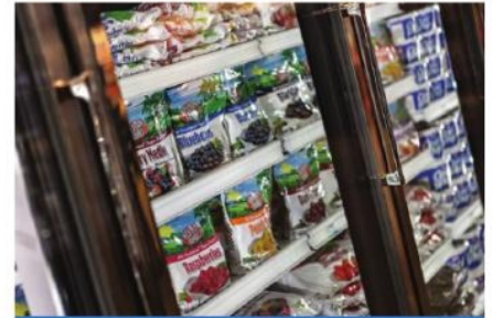
Higher efficiency ECM fans are now used on cases that need a steady air curtain to keep cold air from escaping.
