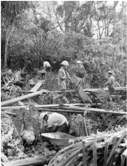
ABOVE / Dangerous excavations: Phosphate miners on Makatea in 1962 cart wheelbarrows loaded with phosphate sand along narrow footbridges spanning deep, limestone-walled pits. PHOTO COURTESY OF LOUIS MOLET / TAHITI HERITAGE
