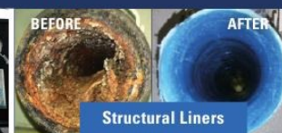
4" Cast Iron Before & After Epoxy Lined
