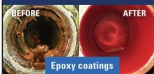
3" Water Main Before & After Epoxy Coated
