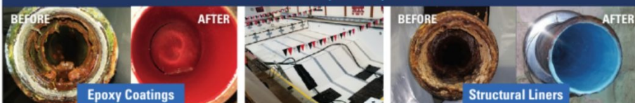
3" Water Main Before & After Epoxy Coated
