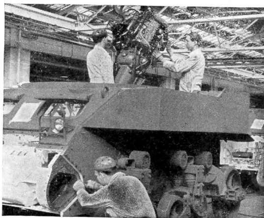
Cadillac engines with Hydramatic transmissions provide motive power for the speedy M-3 tanks and the M-8 howitzer motor carriages.
