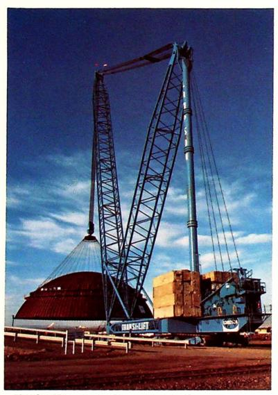
TRANSI-LIFT #1 at Hanford Site 1 walking with 450 ton Dome on the 340' of boom on March 28, 1981. Lampson has delivered two TRANSI-LIFTS to Scotland this year.
