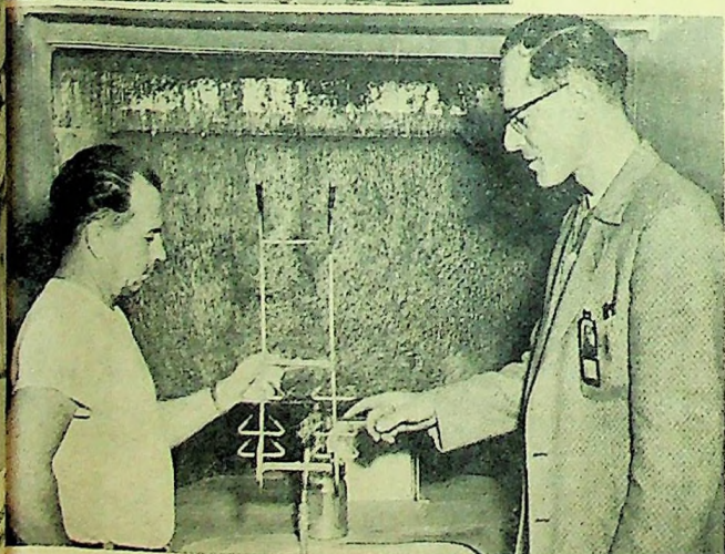
BY A WATERFALL. George Henderson, who mans the paint shop, discusses coating of a metal rack with Jim Berwick, paint estimator. "Waterfall" in background serves to eliminate paint fumes. Mr. Henderson is a specialist in all types of paint coatings and plastic coatings.
