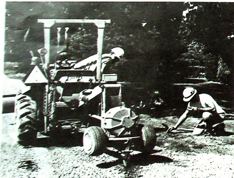
A General Telephone crew buries cable along a Kennewick street after carefully checking the location of an underground water pipe.
