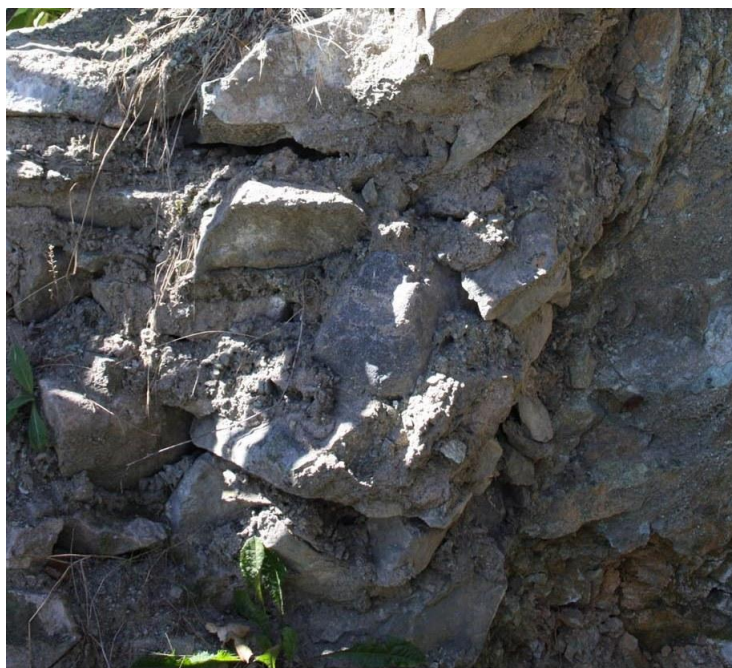
Figure 8: Rock condition at cave entrance (dry condition).
