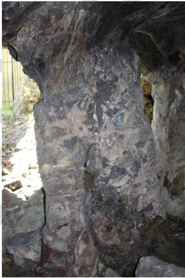
Figure 6: Cave rock pillar showing evidence of spalling
