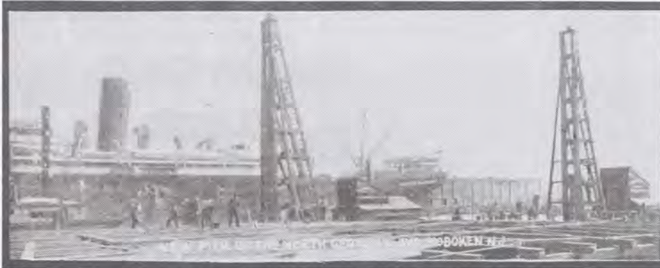
Building the new pier for North German Lloyd.
