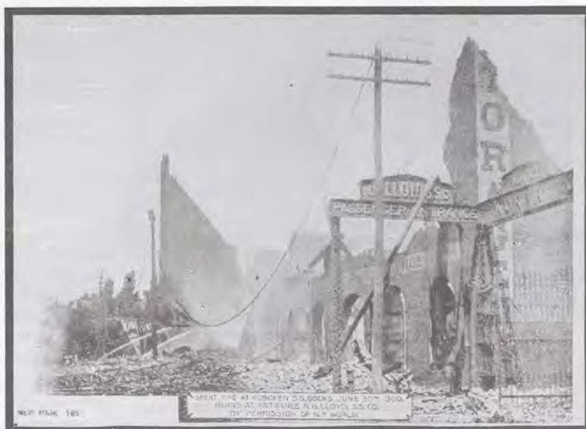
Ruins at the entrance of the North German Lloyd pier, after the fire on June 30, 1900.
