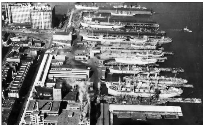
Aerial view of the Hoboken docks, c. 1950, HHM collection.
