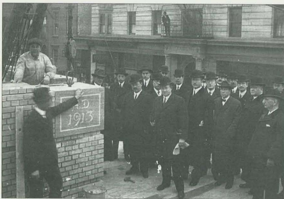
Laying the cornerstone for No. 1 School, now David E. Rue School, 1913. Robert Kirchgessner watches from Third Street.
