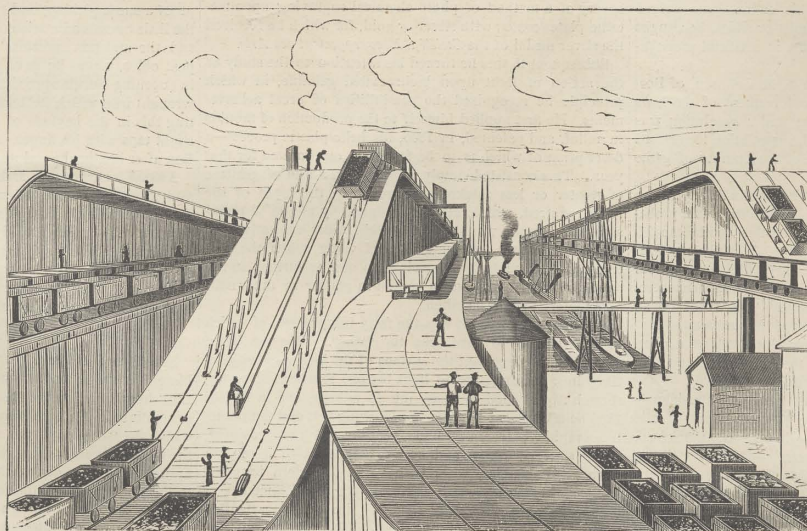
REAR VIEW OF PIERS.—RETURN INCLINE.
