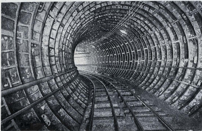
CURVE IN EAST-BOUND TUNNEL AT THE CORNER OF MORTON & GREENWICH STS. TRACKS ARE FOR CONTRACTORS EXCAVATION TRAINS
