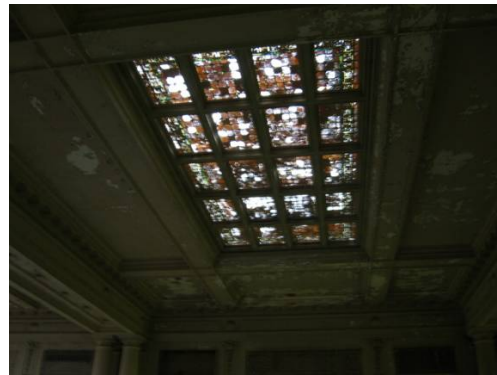
Interior conditions of the Ferry Concourse.
