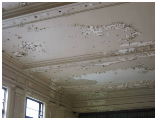
Ceiling of Stepped Concourse.
