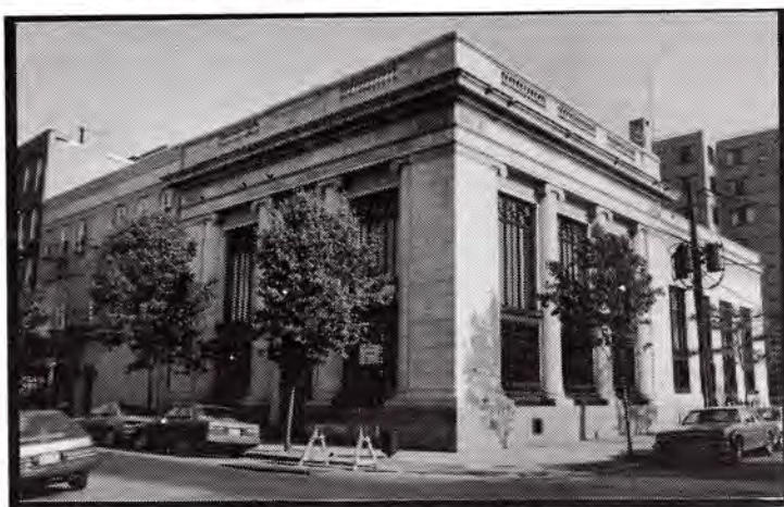
Jefferson Trust Building
