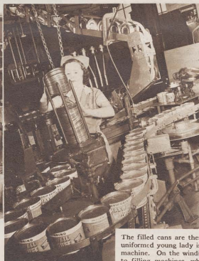
From the granulator it enters the automatic filler shown here. This filling device fills cans at the rate of 85 a minute, and fills them tirelessly and accurately.
