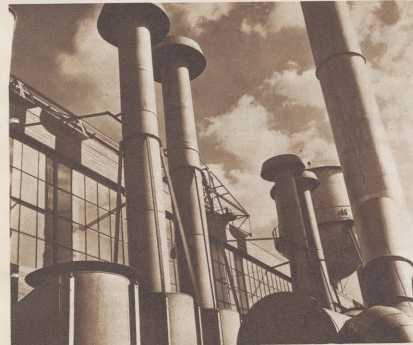
Picturesque sky shot atop new Maxwell House plant—on Hoboken waterfront—shows roof ventilators. Every exhaust from the cleaning and roasting process is protected by dust separators and chaff collector supplied by Jabez Burns.
