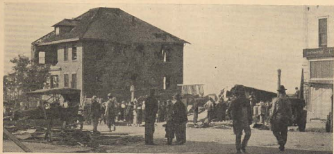
The Hoisington Y. M. C. A. with a Big Hole in the Front Wall and Much Battered Generally
