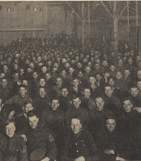
Men at Hudson Hut
