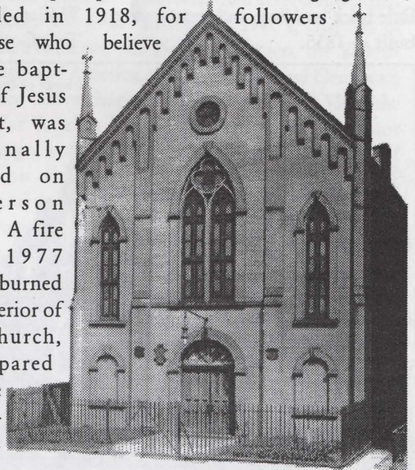
The German Methodist Episcopal Church (ca. 1933) on Garden Street between First and Second streets. At the time, the building was used for the unemployed. (Hoboken Public Library Picture Collection)
