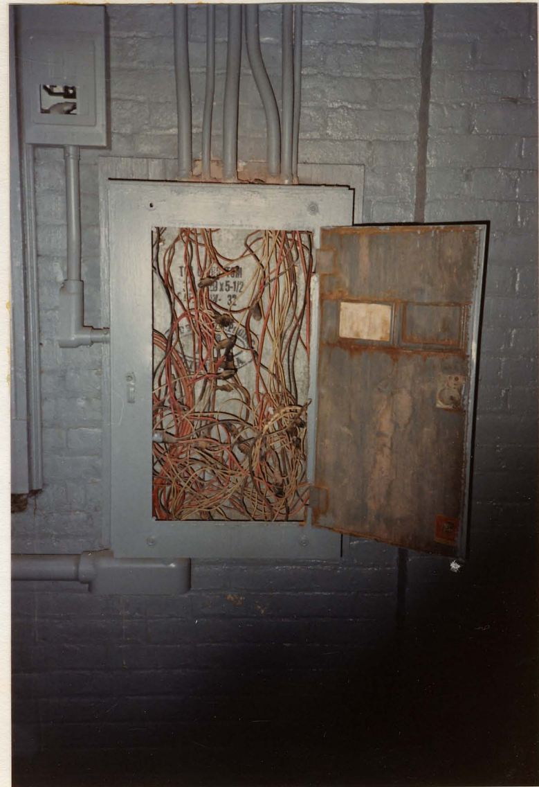
EXISTING ELECTRICAL CONDITIONS
