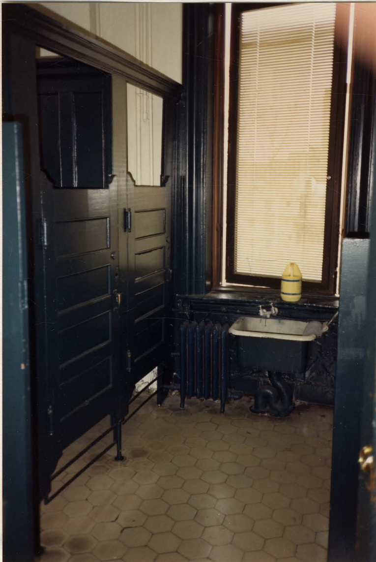
EXISTING TOILET FACILITIES
