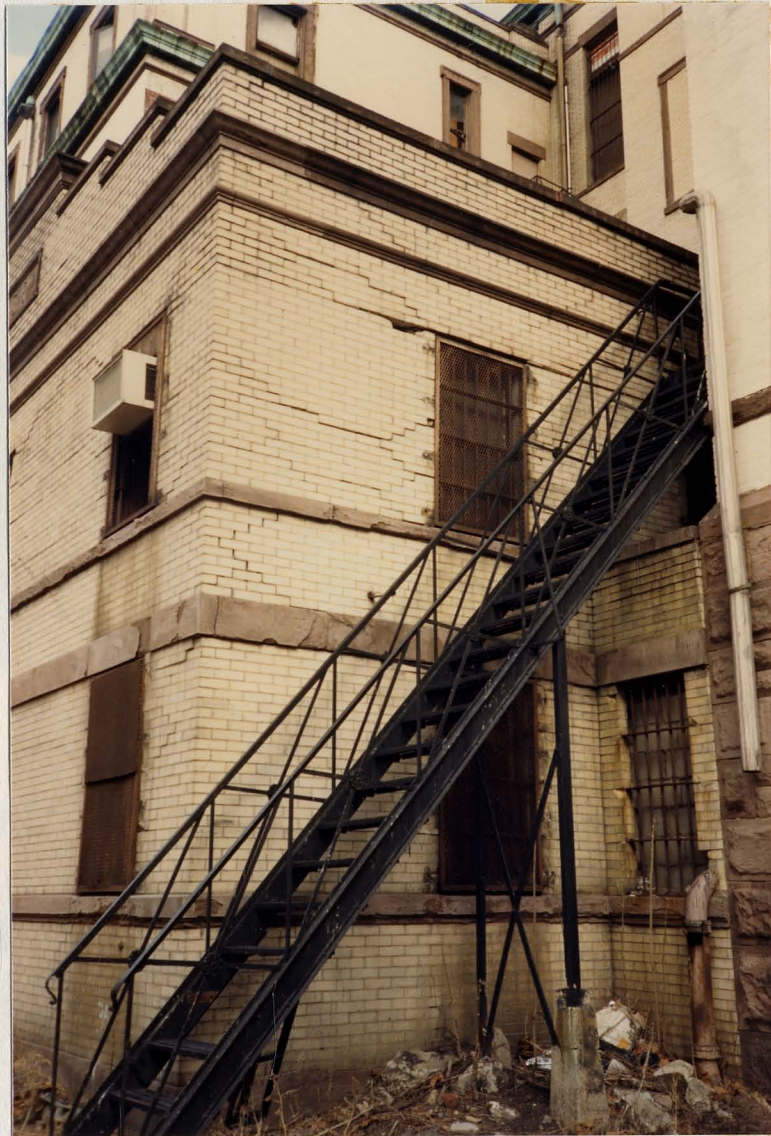
EXISTING EXTERIOR AND FIRE EXIT
