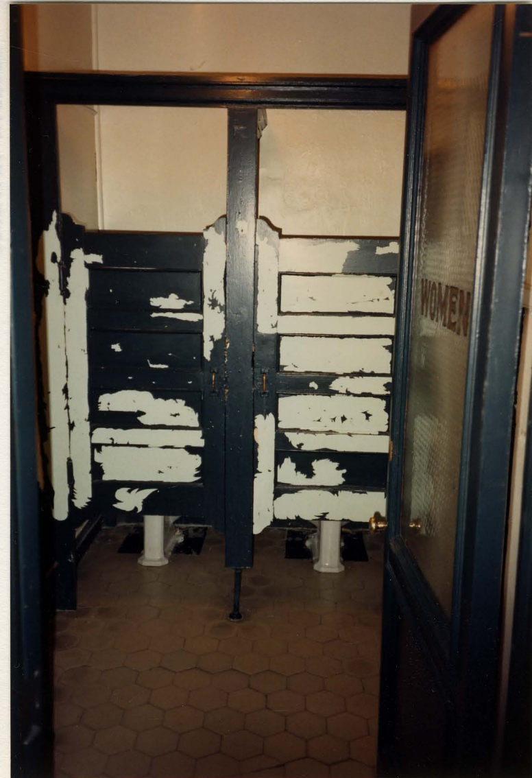
EXISTING TOILET FACILITIES
