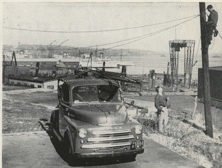
• Rerouting cable into Stevens Tech are Repairmen Joseph Morris and Jim McQuade with the city's busy waterfront making an imposing background.
