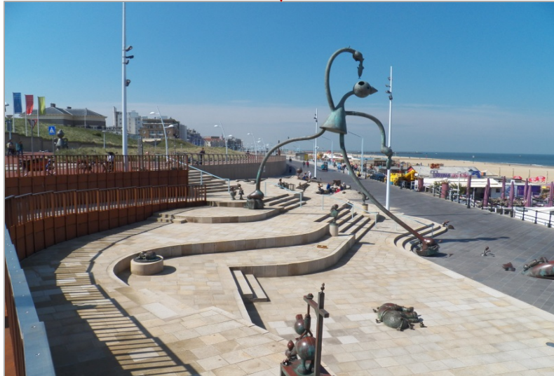
armored levee - Scheveningen, Netherlands
