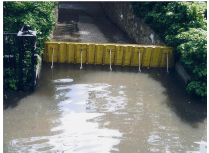
Flood gate floats to deploy automatically without human intervention or power.
