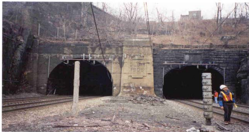
Figure 1 View of East Portals
