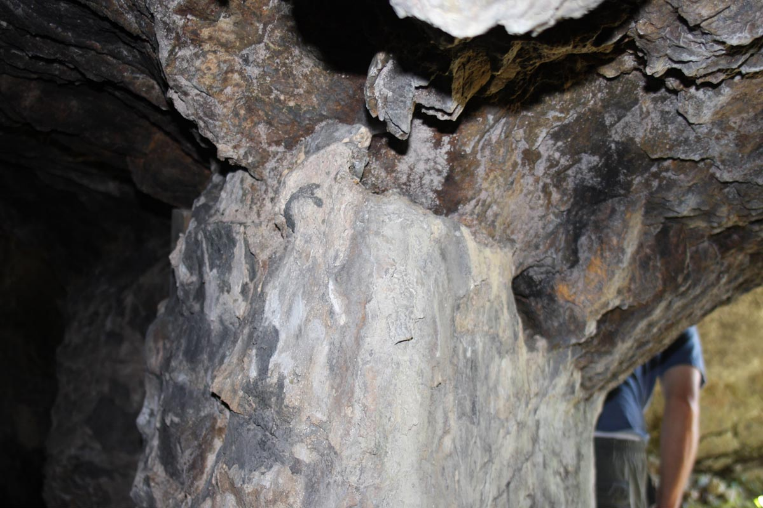
015 Sybil's Cave, Hoboken NJ 9-21-2010 Detail view of the SW pillar near top and ceiling; view is NE of the SW side of pillar
