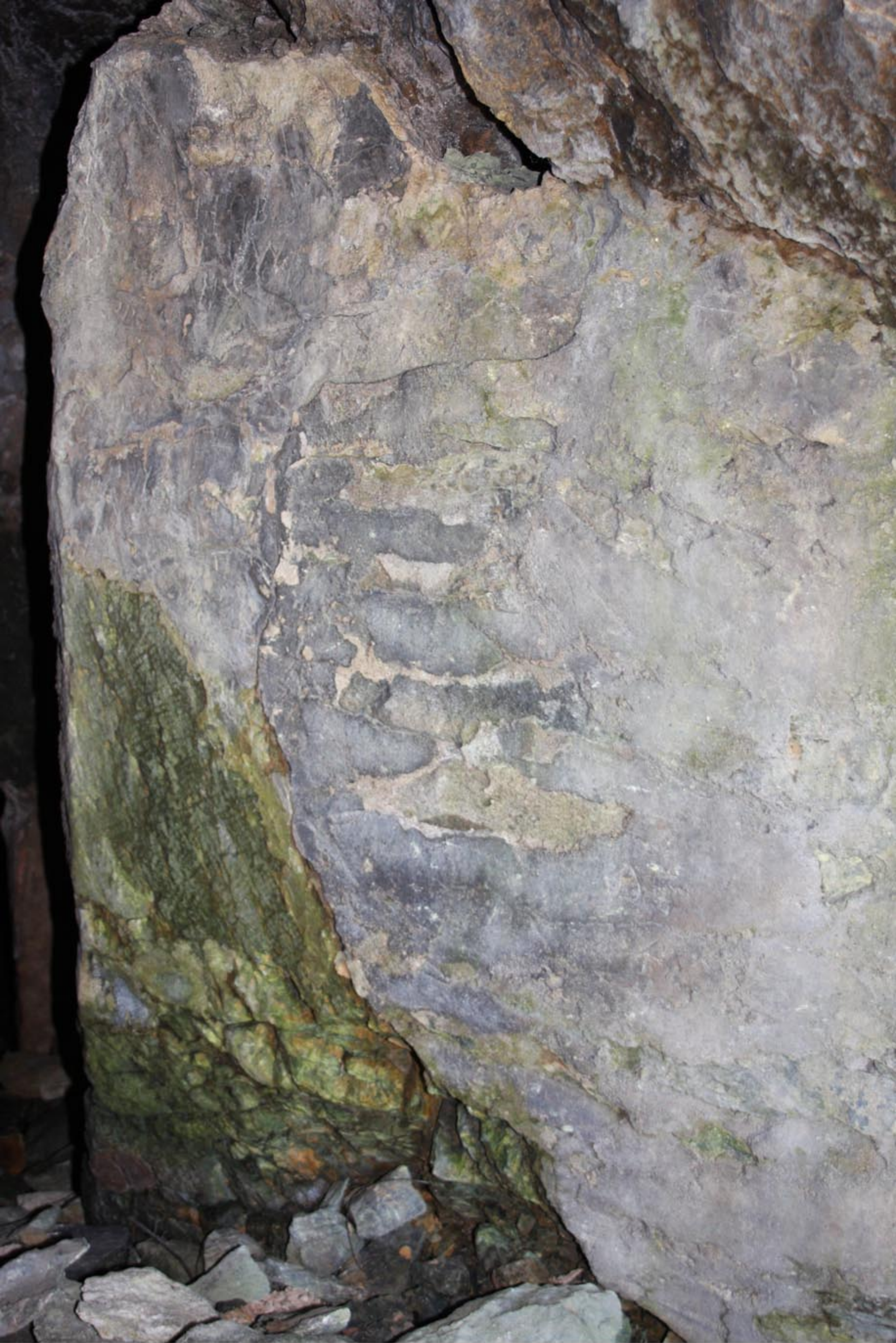
010 Sybil's Cave, Hoboken NJ 9-21-2010 Detail of SE bottom corner of SE pillar
