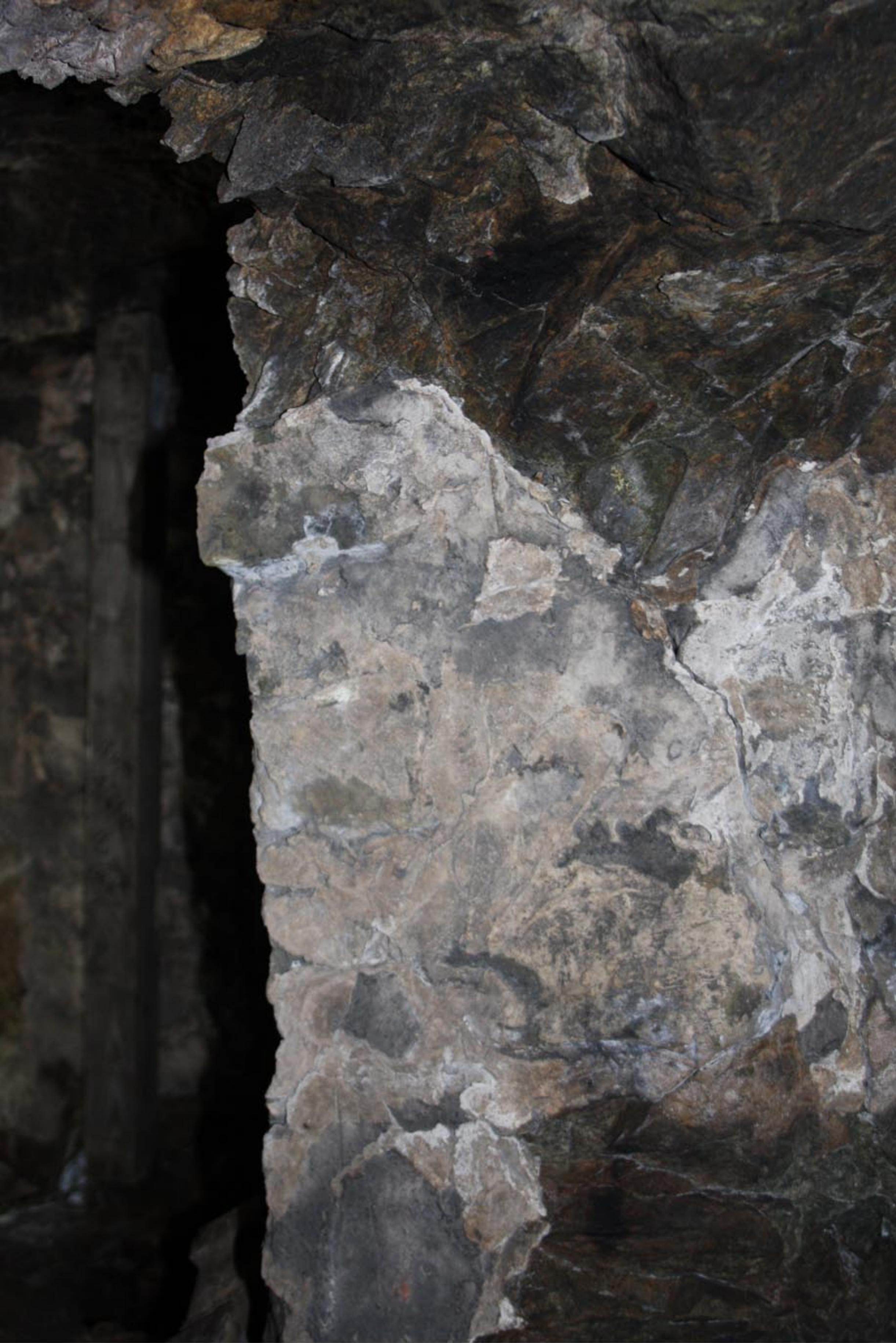
026 Sybil's Cave, Hoboken NJ 9-21-2010 Detail of upper SE corner of NE pillar
