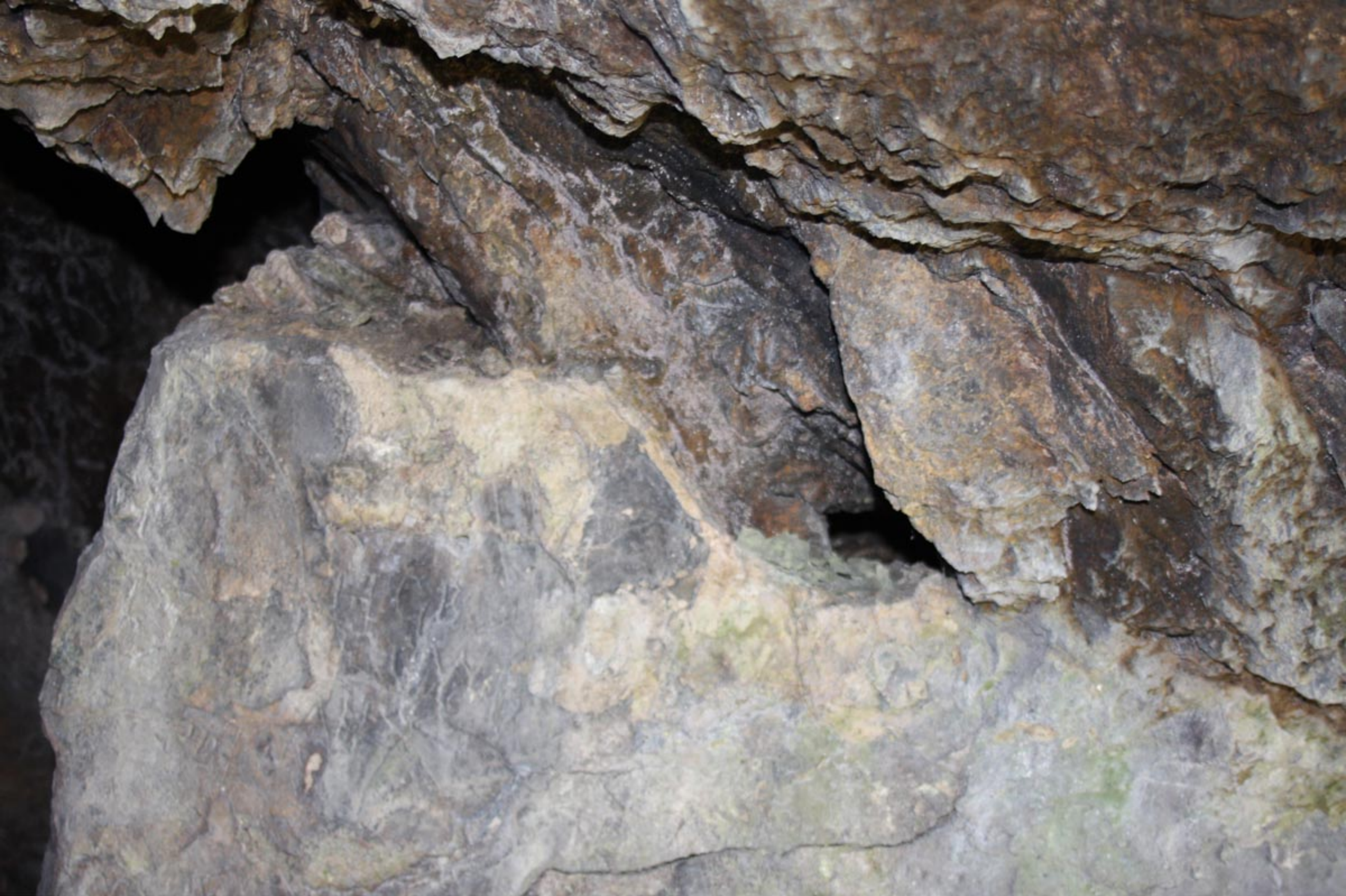
012 Sybil's Cave, Hoboken NJ 9-21-2010 Closer detail of image seen in 011 of SE corner of SE pillar at ceiling
