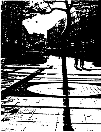
Durable steel, concrete and cast iron grates are carefully selected and integrated with the paving pattern to complement other site furnishings and adjacent buildings. (Munich, Germany, and Camden, New Jersey)
