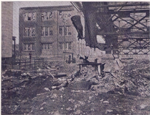
Courtesy of The New York Evening Journal A typical "Peace" argument. On March 31, 1909, six persons were injured and several houses in Hoboken (N. J.), partly demolished by the explosion of a nitro-glycerine bomb placed under a new $350,000 traffic viaduct being built by a construction company involved in labor troubles.
