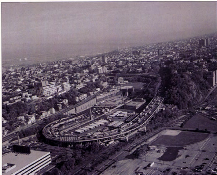
Figure 15: New Jersey Route 3 approach to the Lincoln Tunnel loops its way down from the Bergen Hill. Aerial (1991) from the Library of Congress, Historic American Engineering Record, NY-307.
