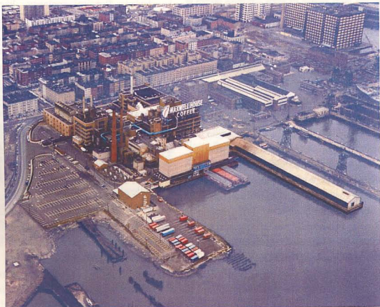
A circa-1990 aerial view of the Maxwell House Coffee Plant (Courtesy Kraft Foods, Inc.).
