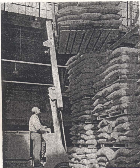
Sacks of green coffee beans await processing in the new Maxwell House Coffee Plant ( Compressed Air Magazine , March 1941. Courtesy Kraft Foods, Inc.).
