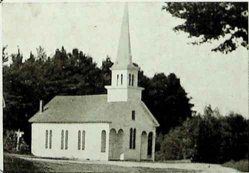
Congregational Church, Kensington, N. H.
