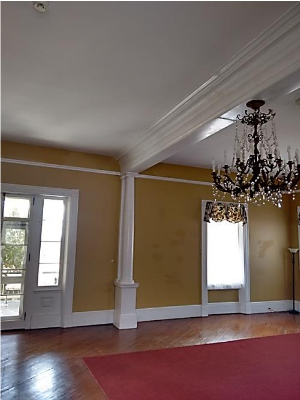
Finished ballroom after the installation of the structural steel beam and columns, wood trim and floor repairs.
