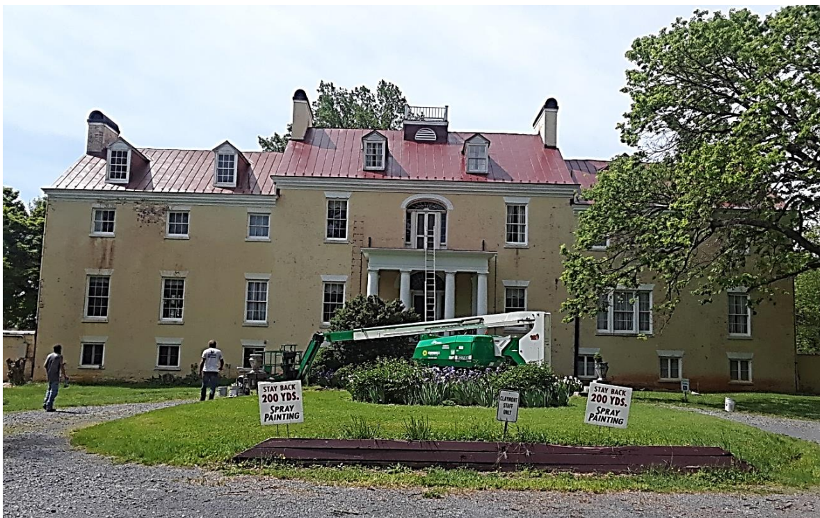
Cleaned, Repaired and Primed Roof
