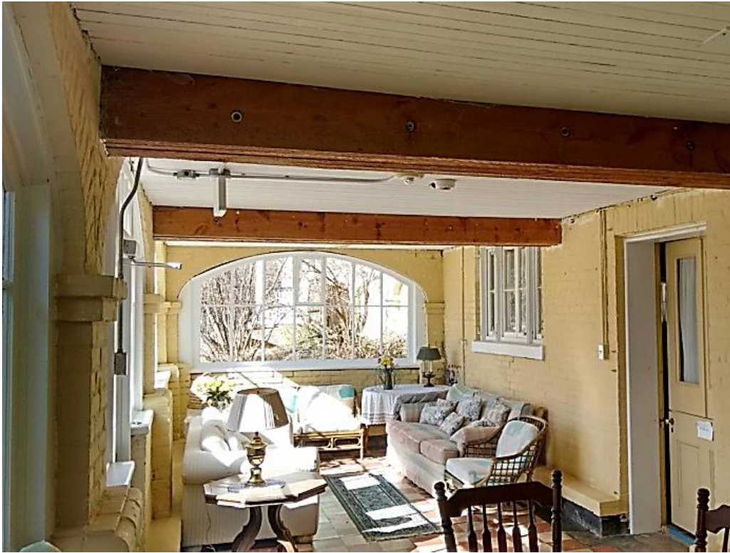
Structural beams supporting verandah and ballroom above
