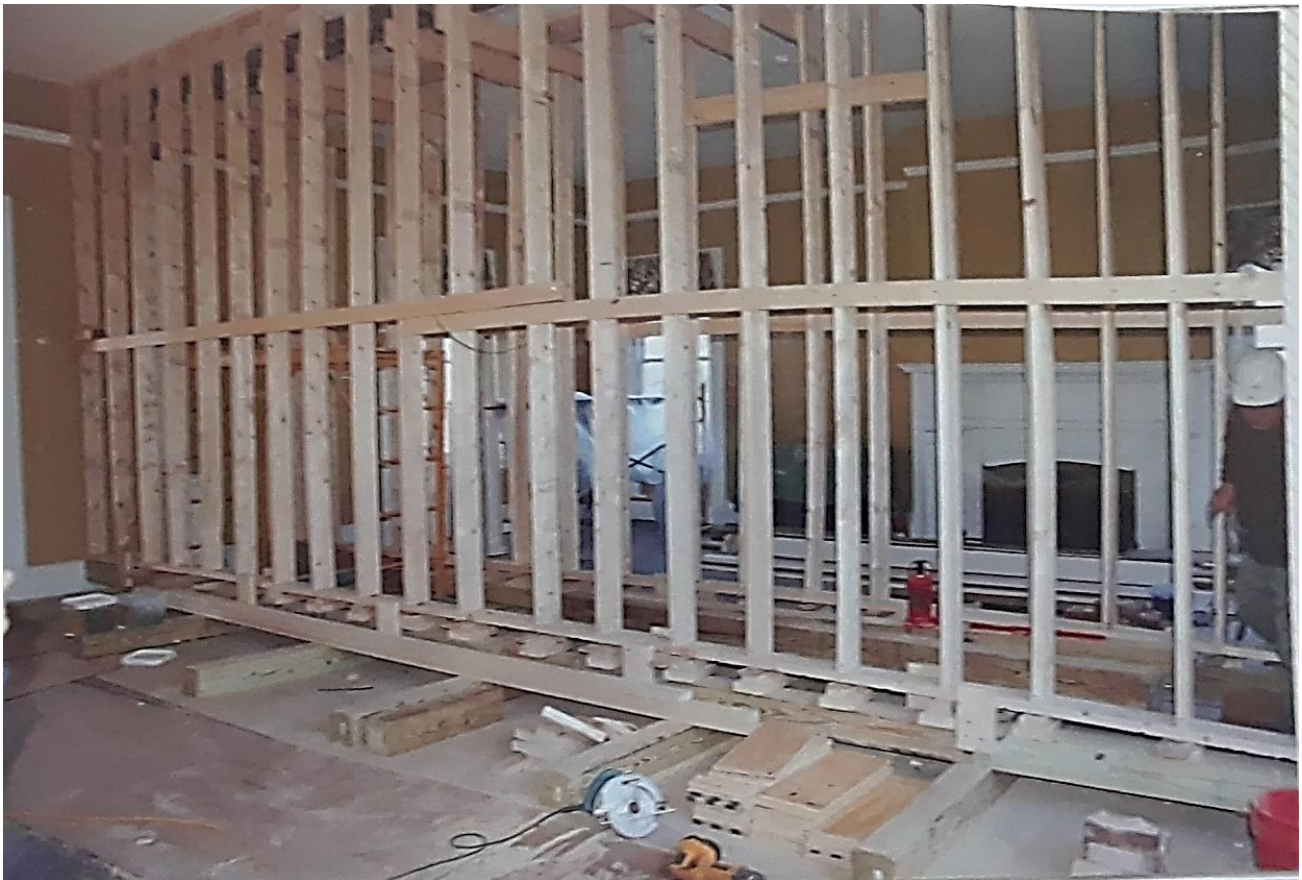
Temporary support to ballroom ceiling during beam installation
