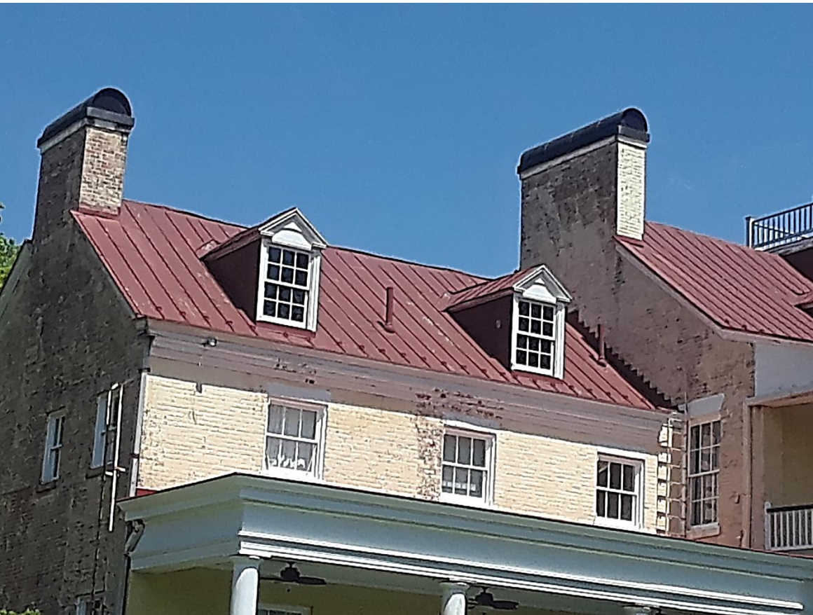
Exiting Roof Conditiona
