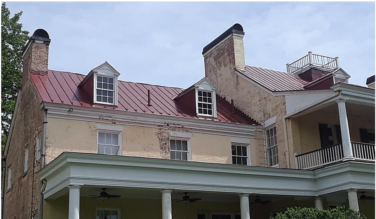
Completed Roof Restoration.
