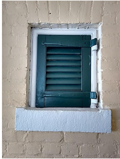
Original exterior window with shutters and hardware from 1890
