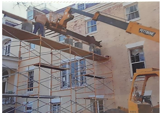
Installation of ballroom ceiling structural support beam
