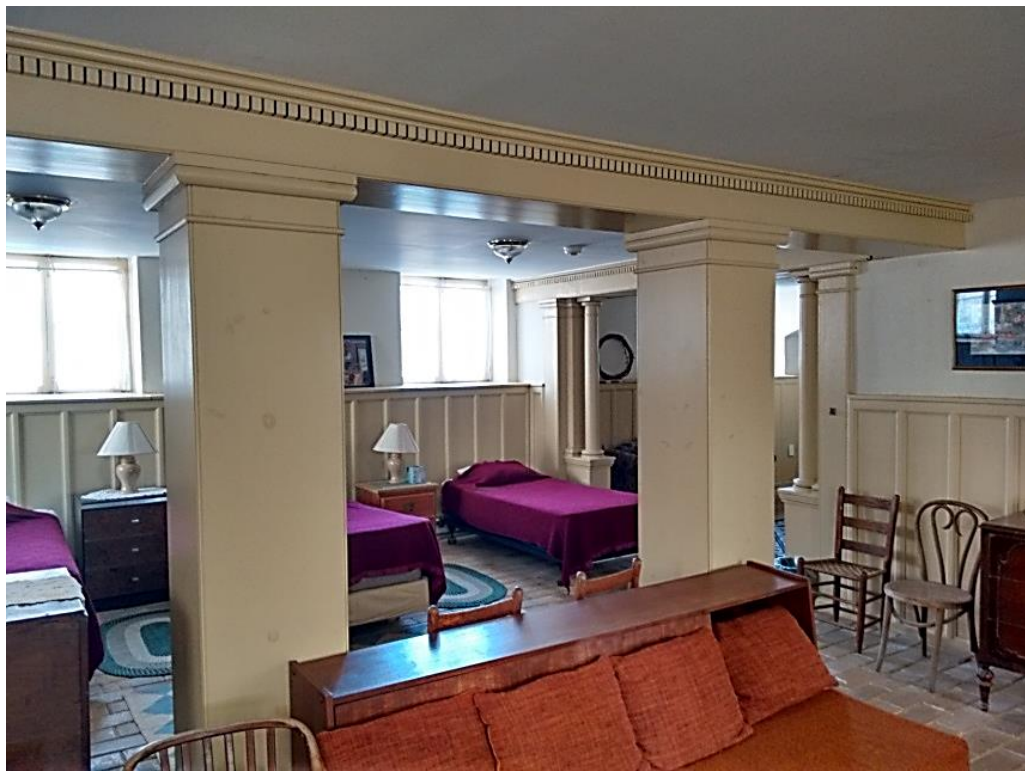
Finished room with wood trim covering the ceiling beam and columns
