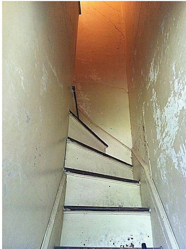
"Secret Stair" from Second Floor servery to Third Floor bedrooms
