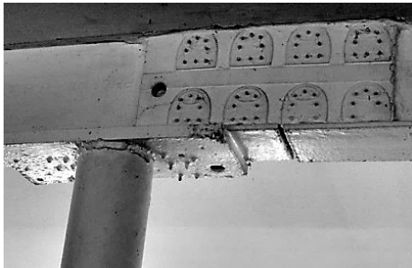
O'Sullivan Rubber metal shoe molds used to weld beams to columns
