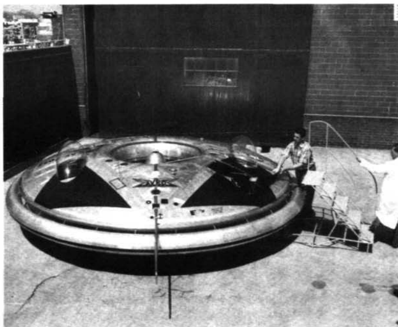
Photograph, formerly classified "secret," of the Avrocar Test Vehicle. Its first untethered flight, November 12, 1959, revealed serious instability problems that were never solved.
