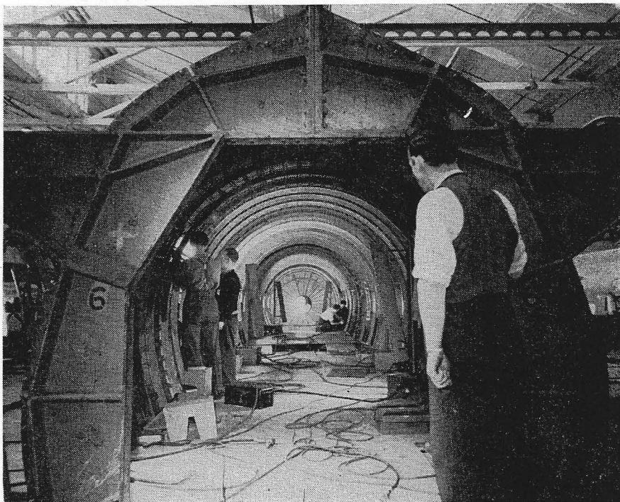
RIGHT UPPER: The first of 22 four-engined Canadair Fours on the final assembly line. The fuselage has been joined to the centre wing section.
